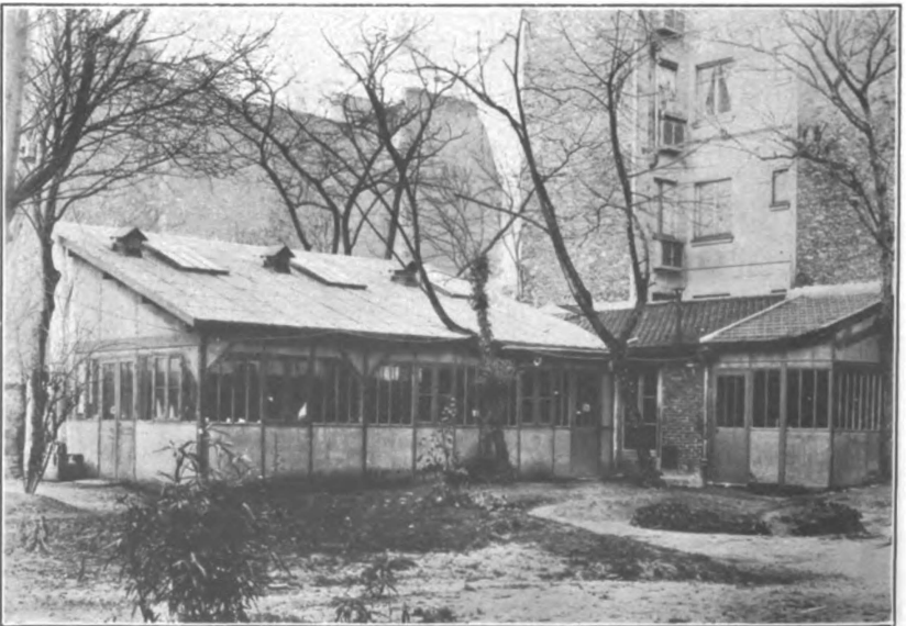
REAR VIEW OF RESEARCH AND INSPECTION LABORATORY. PARIS, FRANCE.
