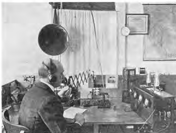
STATION "22L," LOCATED AT VALLEY STREAM, L. I. USING TWO 50-WATT RADIOTRONS, THIS STATION HAS BEEN HEARD OVER 1,900 MILES OVERLAND
